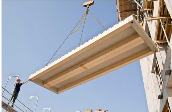
Photograph 2: Timber concrete composite floor panel
