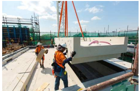
Photographs 8 and 9: Precast geopolymer beams installation
