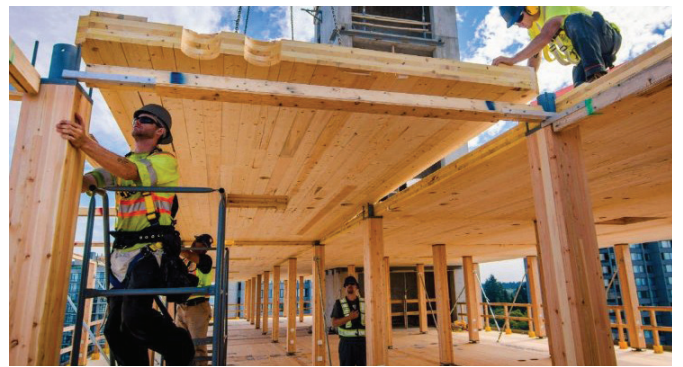
The 18-storey Brock Commons in Canada (see cover image) was erected in 9.5 weeks by nine men
