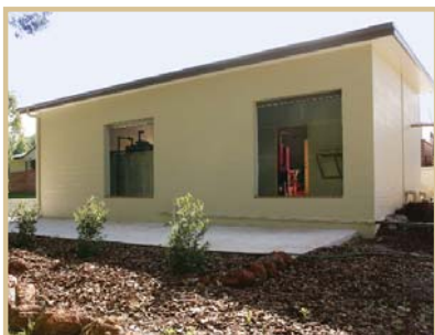
This decentralised wastewater treatment plant allows a residential development to be self sufficient in water and wastewater services.
