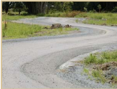
Gravel edge – Site roads have been designed to minimise hard kerbs and drainage and to make best use of the natural setting and existing vegetation.
