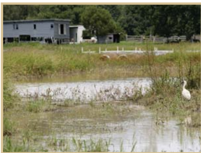
The stormwater swales provide a natural environment for water quality control and for birdlife as well.
