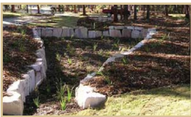
Managed stormwater runoff uses swales and bioretention filters
