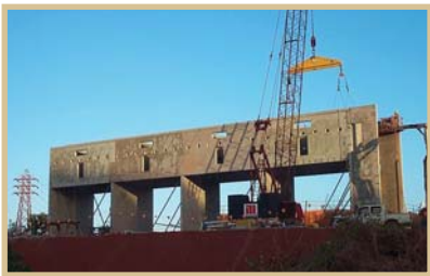
Lifting the precast panels into place and bolting the tower together
