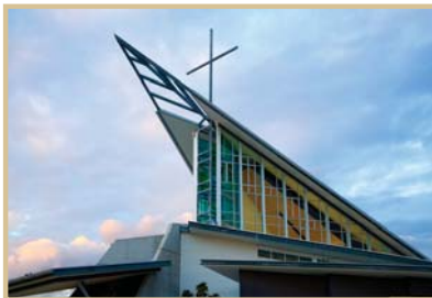
Soaring steel frames sustain glazing
