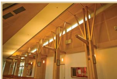
Laminated timber columns brace the high walls
