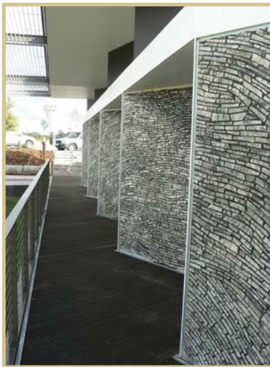
Stone cladding on the steel frame of the Interpretive Centre
