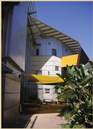
Rear courtyard of main building
