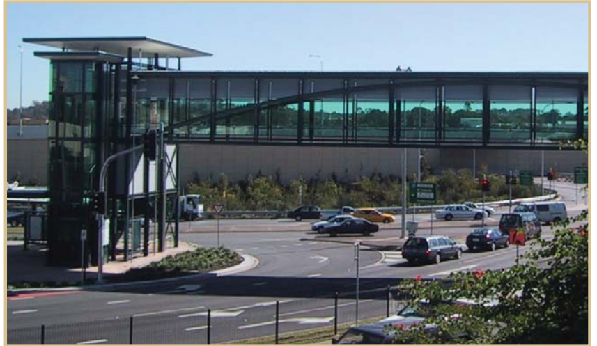
Springwood Bus Station – glass clad & using very light steel combines aesthetics with function
